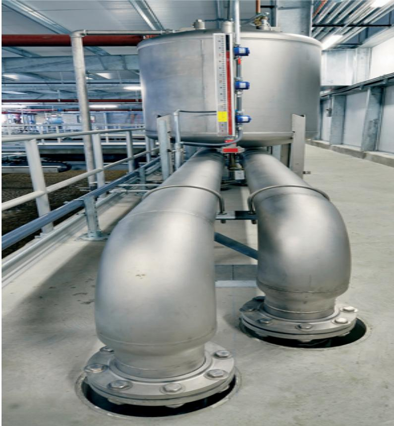
**Variable-flow software lowers costs by automatically regulating flow into the dissolved air flotation tank through dual saturators** Photos: CDM
