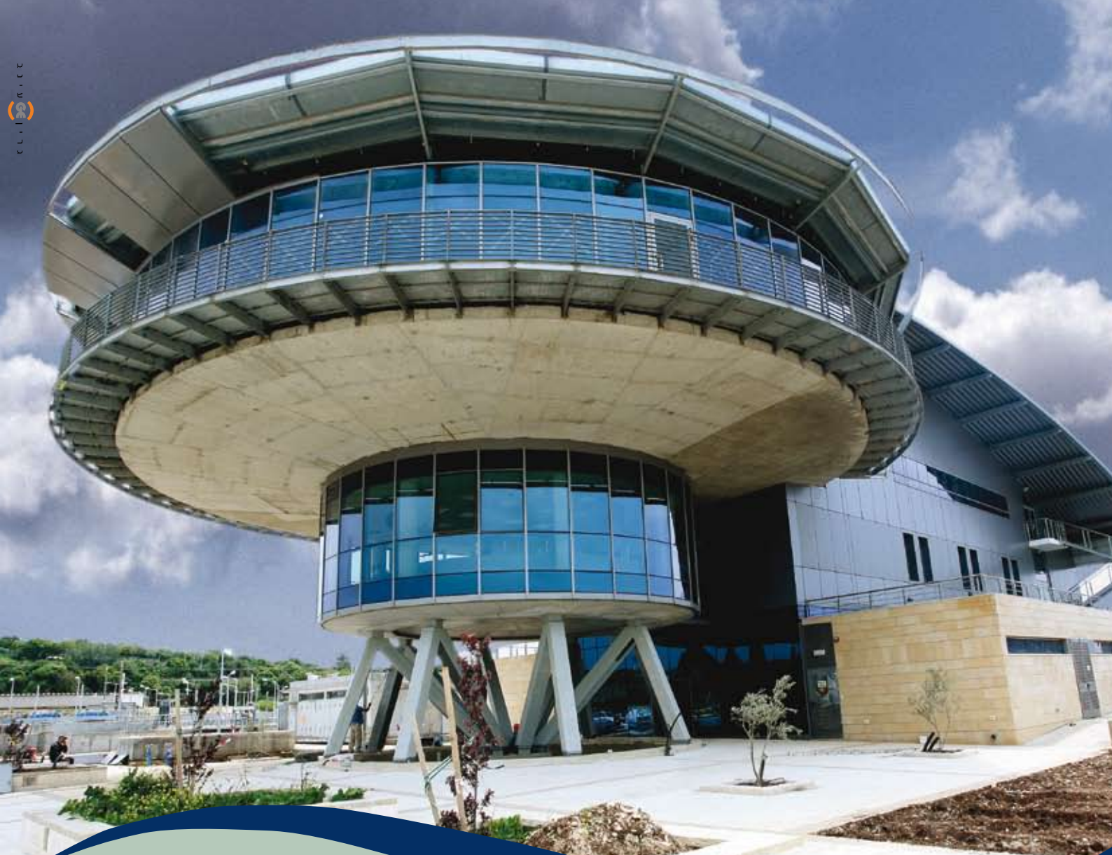
Control Room and Visitors Center. Photograph: Mosh Shai
